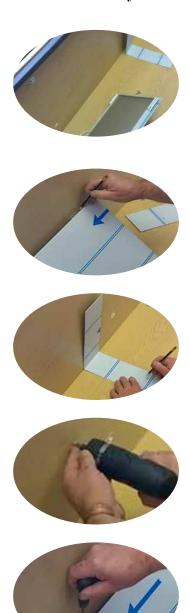
In order to mount in a corner, IHP320a and IHP160a panels have C brackets attached to the 2 long sides of the panel. To install the panel, four mounting screws must be screwed into the wall or desk. The panel is then slides over these screws.
